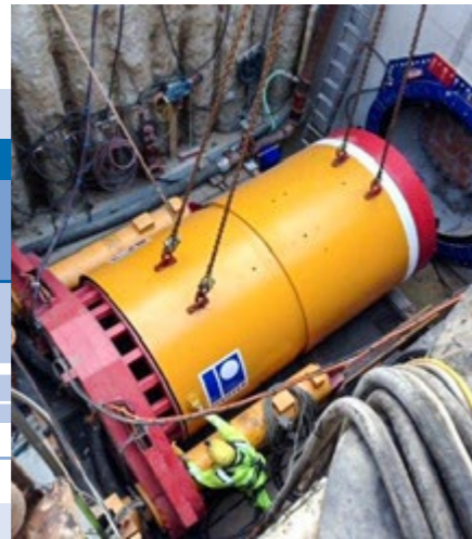
Anbohren Initial drilling
