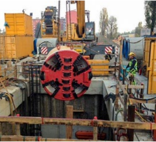
Ablassen der Maschine in den Startschacht Lowering the machine into the entry shaft
