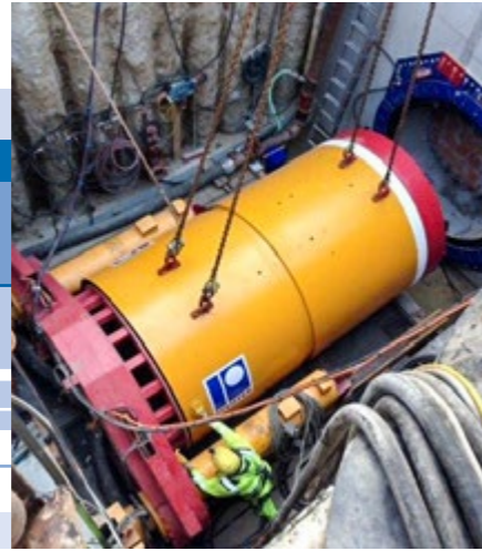
Anbohren Initial drilling
