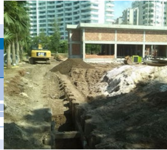
Tece Pumpstation im Bau Tece Pump Station under construction
